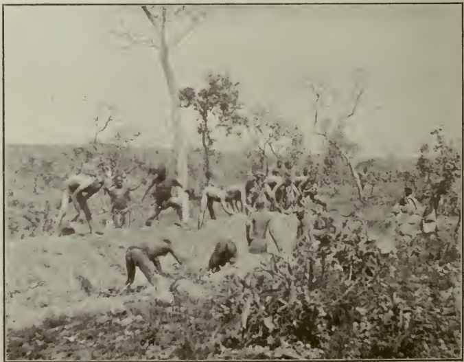
193 NARAGUTA. CONSTRUCTION OF LEAT BY RUKUBAR PAGANS
